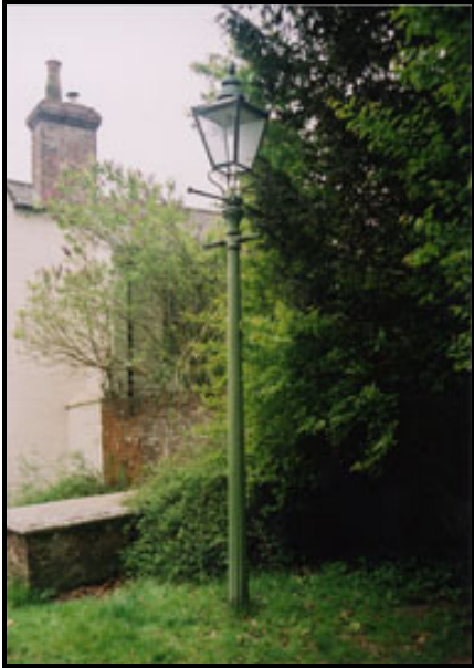
Photo 16: Traditional cast iron street light in the churchyard
