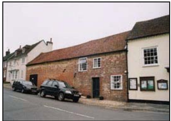
Photo 33: The former barn in High Street has inappropriate windows
