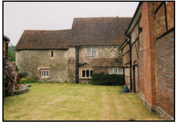
Photo 18: Rear wing of Manor Farm House
