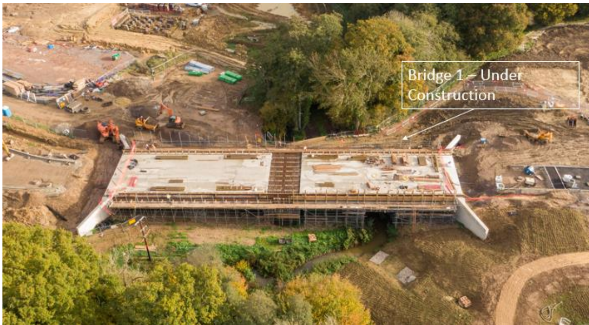
Plate 7: Bridge 1 Progress @ 31 Oct 2020
