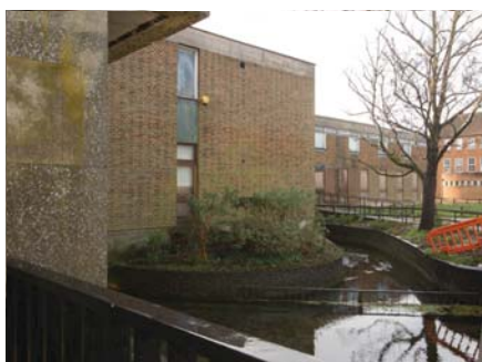
Purchase of Friarsgate medical centre for refurbishment
