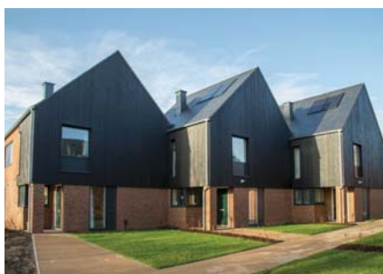
Completed homes at Abbotts Barton
