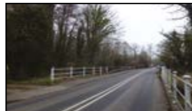
B3335 Highbridge Rd River Bridge
