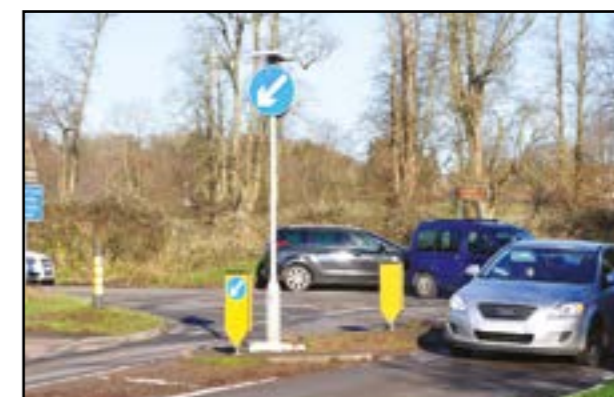
Safe Crossing Point at Highbridge
