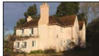
Woodcroft Cottage, Bishopstoke Lane
