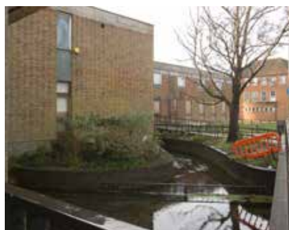
Purchase of Friarsgate Medical Centre as part of Central Winchester Regeneration
