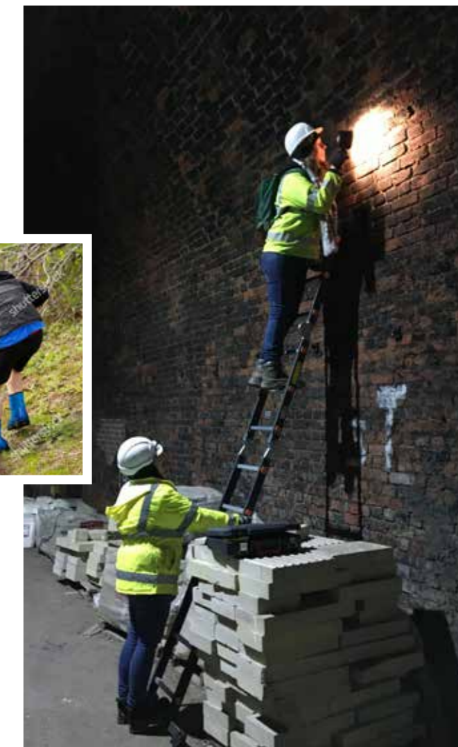
Chesil Tunnel bat roost checks ©Richard Smith
