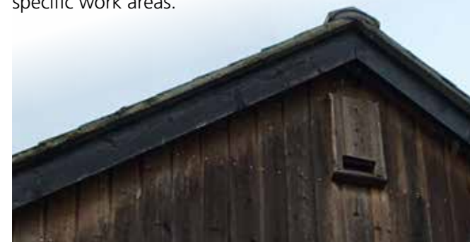
Bat box installation on a new home ©Richard Smith
