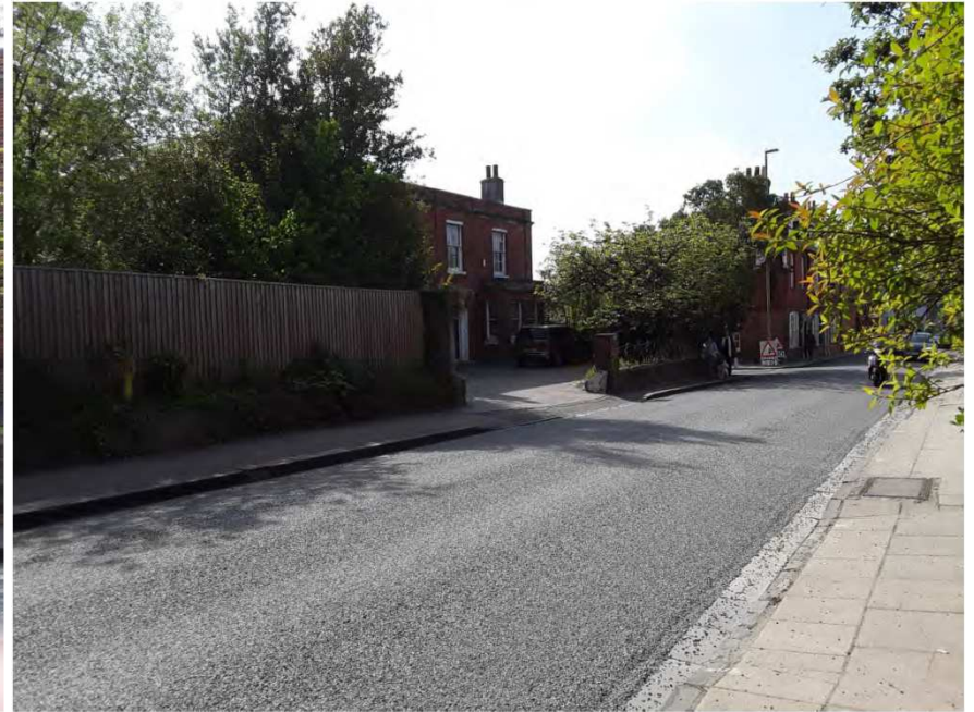
Photo from St Cross Road showing boundary wall of Goodworth House
