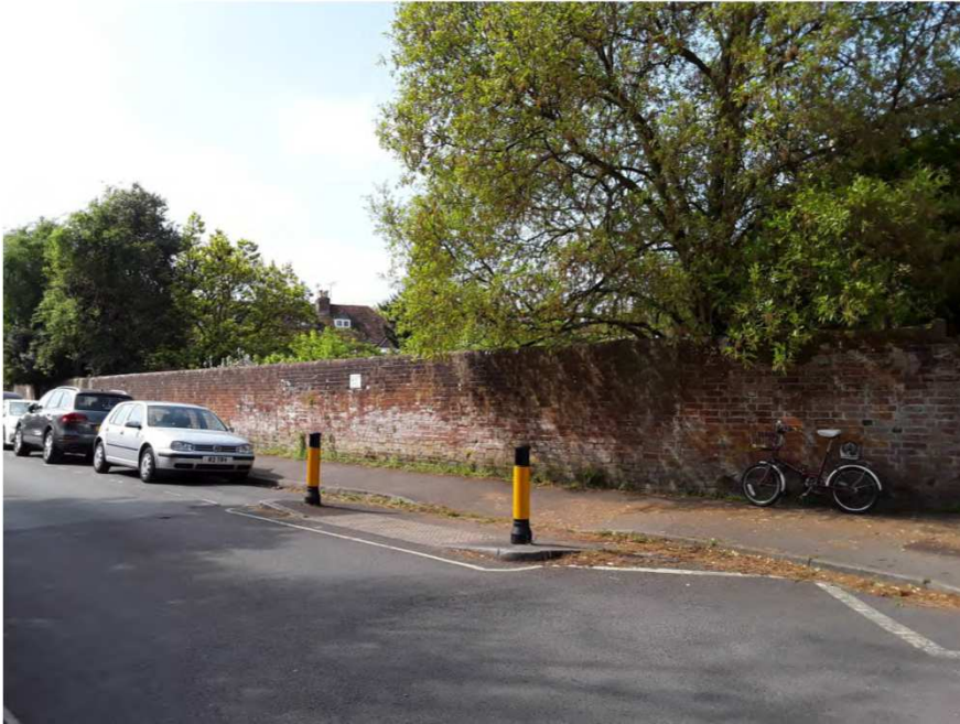
Photo of rear boundary wall on St Faiths Road
