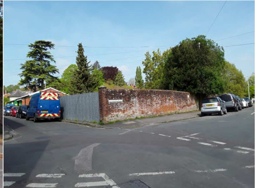
Photo of rear/side boundary wall from St Faiths Road/Cripstead Lane
