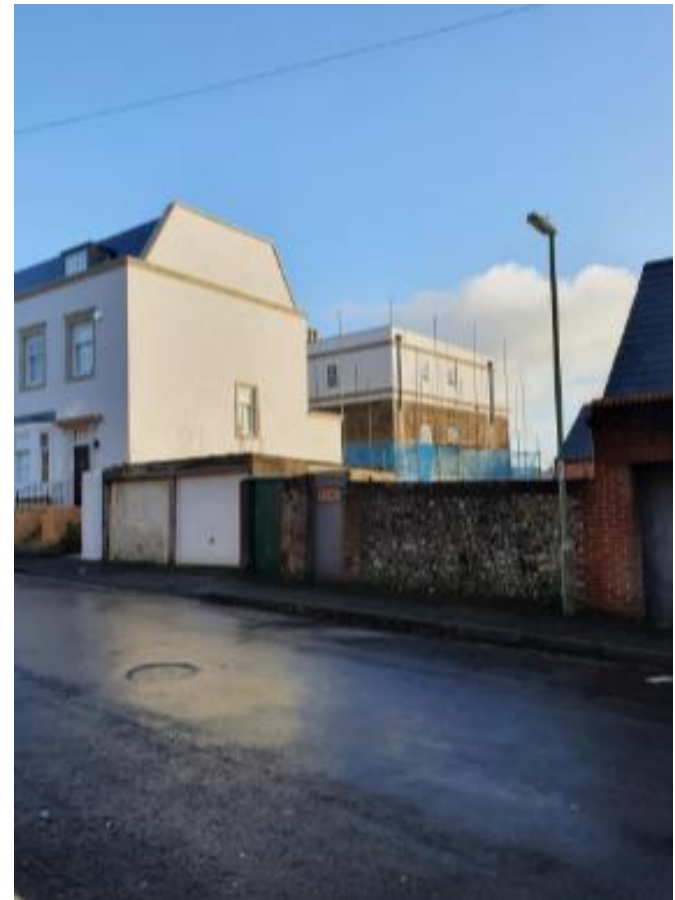
VIEW FROM THE SOUTH- WEST
