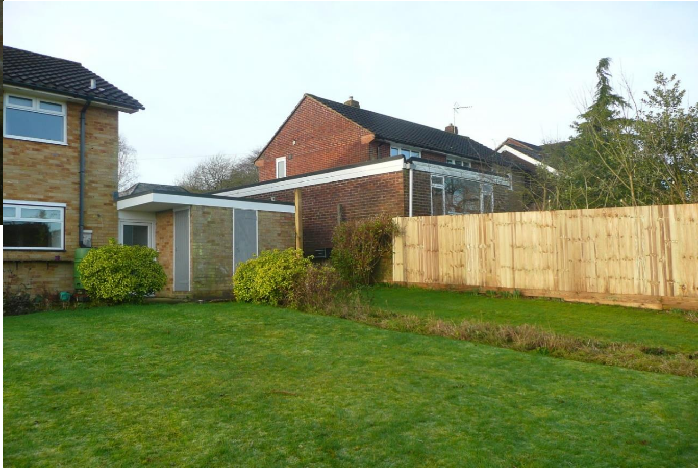
View of the rear of 114 Teg Down Meads from the garden of 112.
