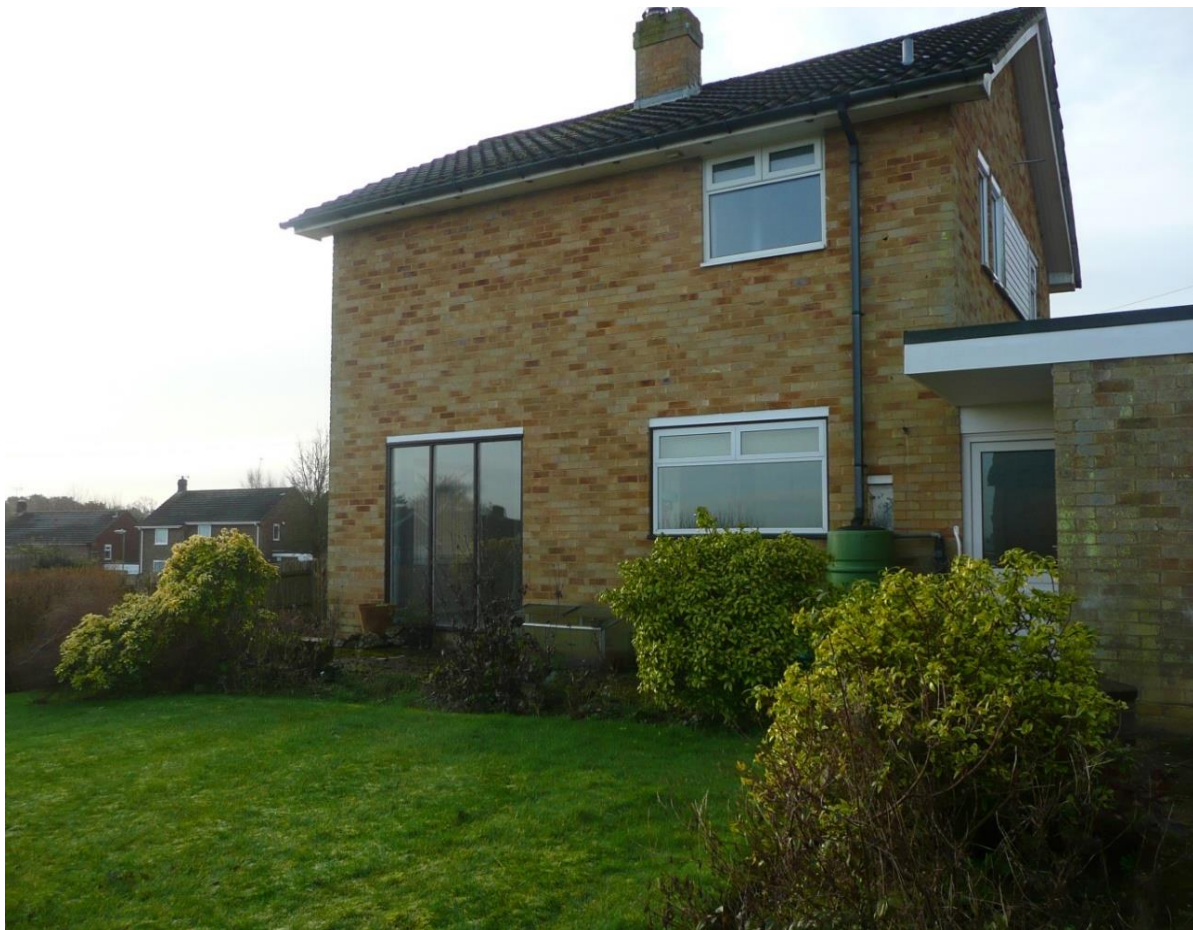
View of the rear of 112 Teg Down Meads
