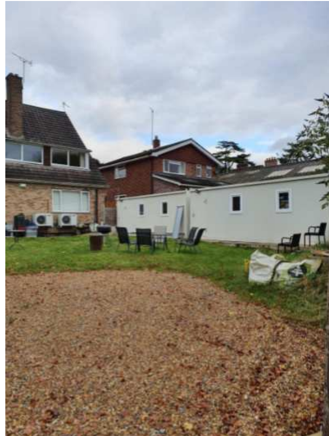
TEMPORARY OUTBUILDING AT REAR VIEWED FROM SOUTH-WEST
