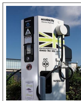
Example of Pod Point 50kW Ecotricity rapid charger
