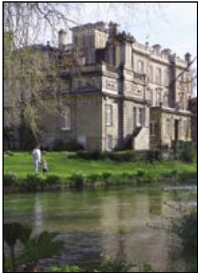
Brambridge House, Kiln Lane
