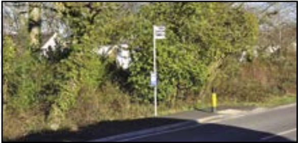
Safer Bus Stop, Church Lane
