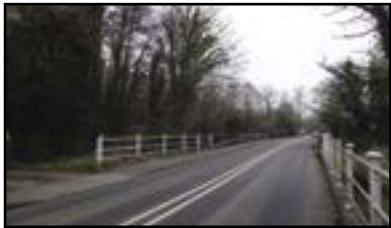
B3335 Highbridge Rd River Bridge
