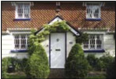
Keepers Cottage, Church Lane
