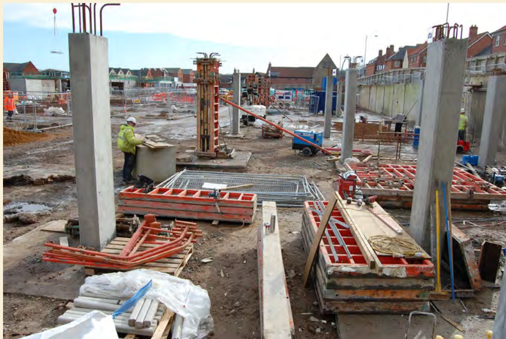
Plate 3: Columns to support a podium slab at St Anne's Quarter in Norwich. Much of the existing slab on the site was retained as the base for the floor of the underground car-park
